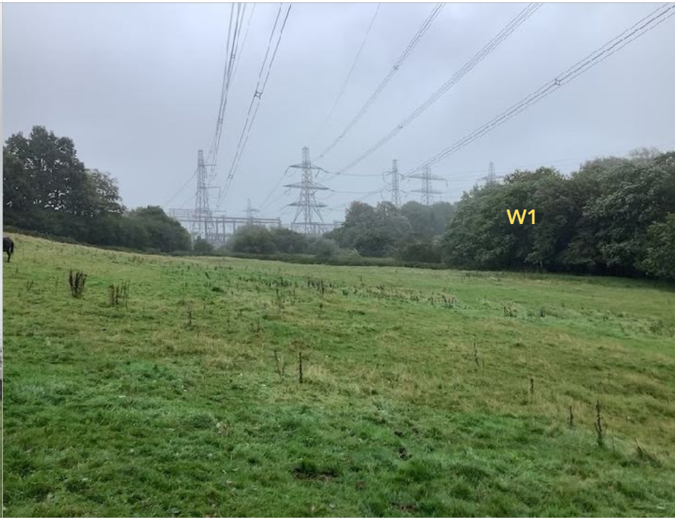
IMAGE 2: View looking north east toward Cilfynydd electrical sub-station.
